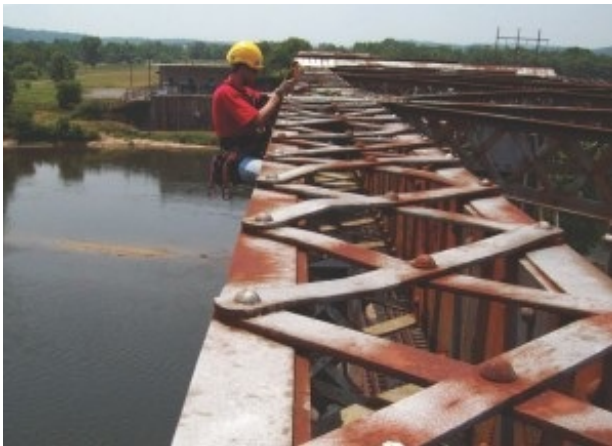
Steve Hobbs, structural engineer for the USACE St. Louis District and level I rope
