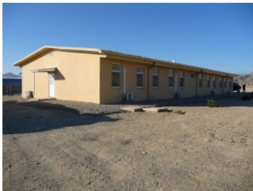
A new office and barracks building for the Afghan fire department at the regional training center at Camp Parsa, Khost province, Afghanistan, was designed to suit Afghan tastes and practices. So far this year, deployed Corps service members and civilians have been working hard in partnership with other agencies to help provide the basics to the war-torn country; USACE continues infrastructure projects valued at nearly $2 billion.
